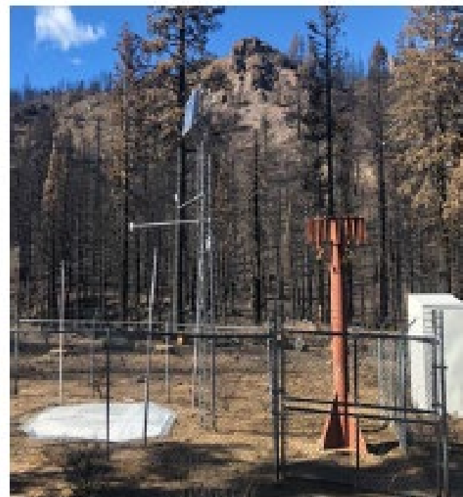
Spratt Ck SNOTEL after rebuild
